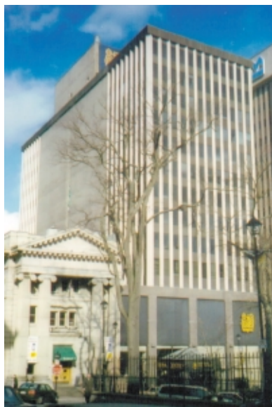
Figure 2 – Royal Bank Building in Halifax
